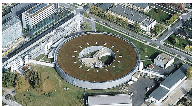
Figure 33. BESSY II in Berlin-Adlershof.
